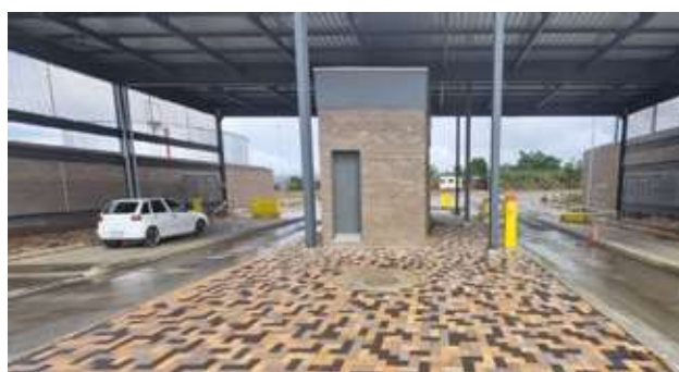
Gaurd House construction done by SMME
