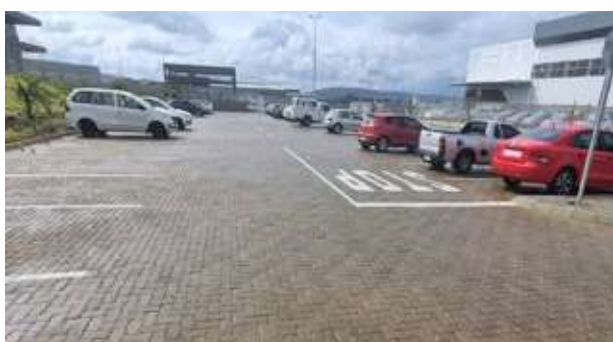
Paving construction done by SMME
