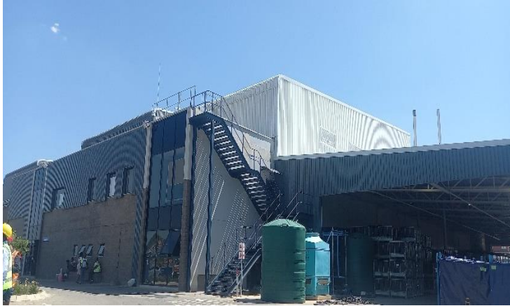
Aeroklasduys Building, Exterior View
