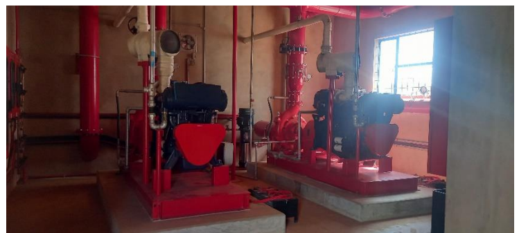
Fire Pump Station: Phase 1.
