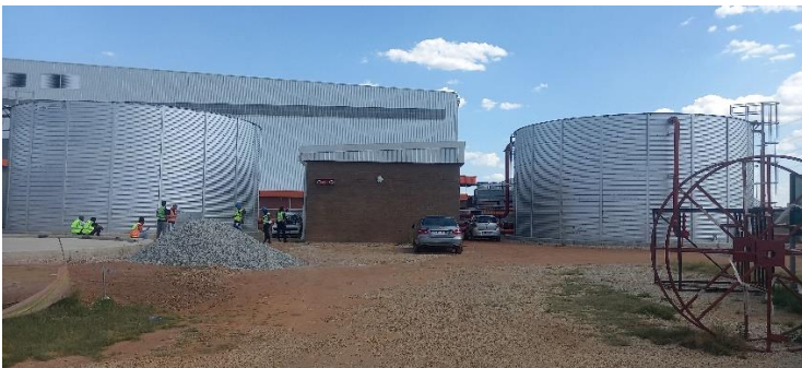
Fire Pump Station: Phase 1.
