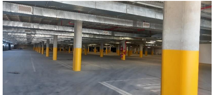
ALSO Building, Basement.
