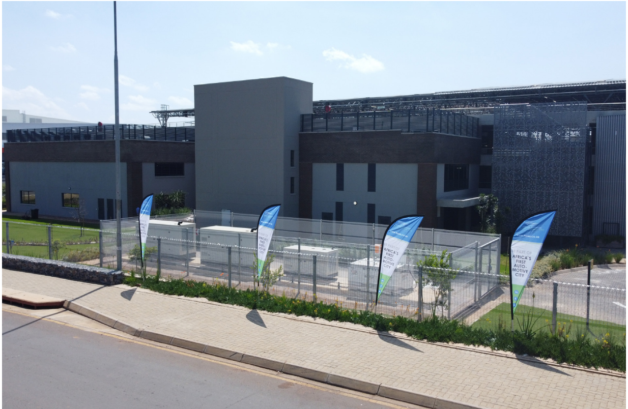
Phase 1 – Central Hub 2024/2025
